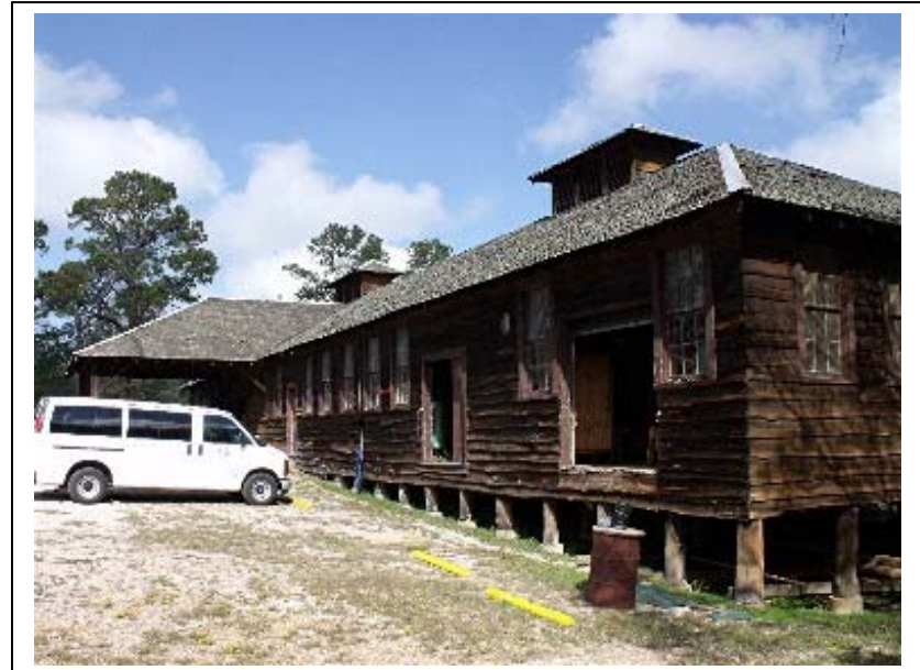
A side view of the Bastrop State Park Historic Shop Building
